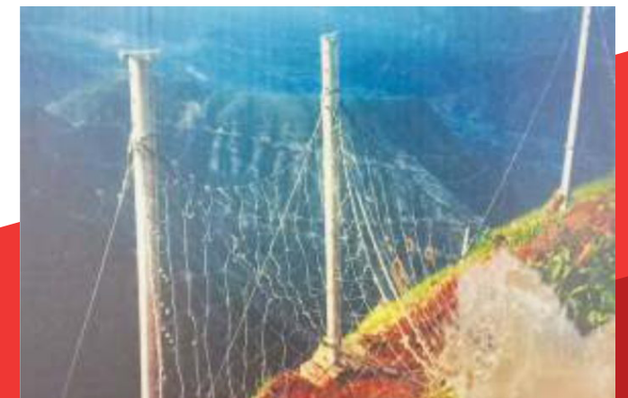
SNOW NETS ASSEMBLY - SNOW AVALANCHE CONTROL STRUCTURE
